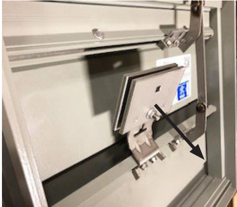
Bend counterweight mounting bracket away from blades.
