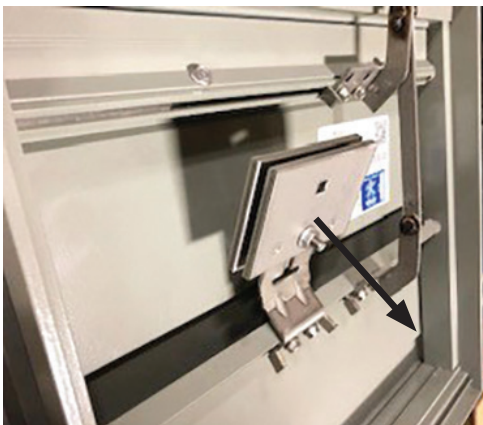
Figure 1: Bending counterbalance bracket away from blade towards the bottom (sill) of damper.
